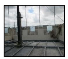
They are now working on the south face of the Tower. The whole of the area where the clock is has been taken back by a complete course of stones. There is also a bad crack to the depth of about 500mm and this will all be repaired.
