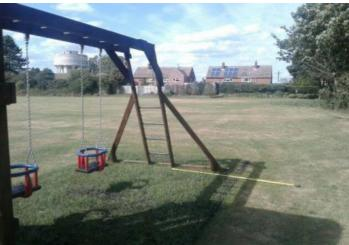
**Finding:** The surfacing dimensions do not meet with the requirements of the current applicable standard
