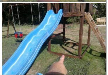
**Finding:** The lower framework forms a hard object within the impact area of the equipment in contravention of the requirements of BS EN 1176 Part 1
