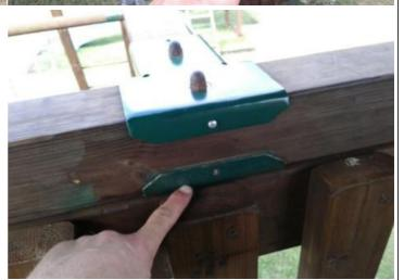
Finding: There is or are fixings missing on the monkey bar Action: Replace all missing fixings connections
