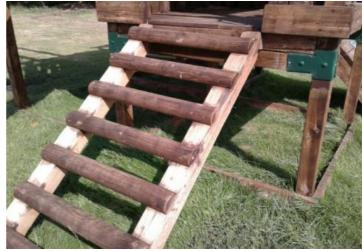
Finding: The item fails to meet the requirements of BS EN Action: Remove the entrapment 1176 Part 1 4.2.7.2 for head and neck entrapment in the access point
