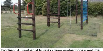
**Finding:** A number of fixing(s) have worked loose and the crossbeam rotates unexpectedly
