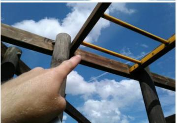
Finding: The item fails to meet the requirements of BS EN Action: Monitor - No remedial work recommended 1176 Part 1 4.2.7.2 for head and neck entrapment in the monkey bars
