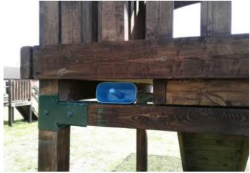
Finding: The item fails to meet the requirements of BS EN Action: Remove the entrapment 1176 Part 1 4.2.7.2 for head and neck entrapment in the framework beneath the platform
