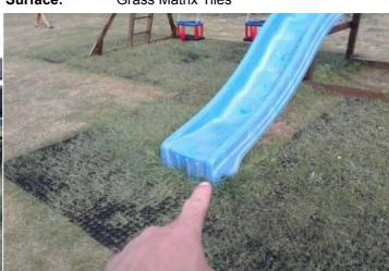
Finding: The slide run out is not secured to the surface
