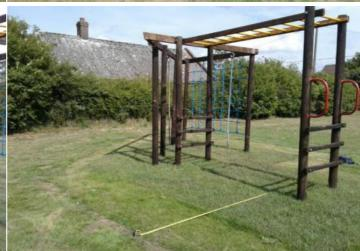
**Finding:** The surfacing dimensions do not meet with the requirements of the current applicable standard (2.32m required/ 0.60mm provided)
