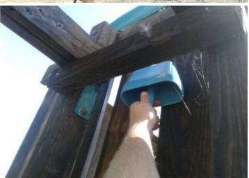
Finding: The item fails to meet the requirements of BS EN Action: Remove the entrapment 1176 Part 1 4.2.7.2 for head and neck entrapment in the monkey bar framework
