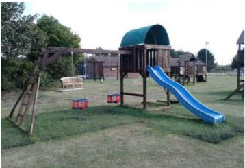
**Finding:** There is/are finger entrapment/s in the platforms and the item fails to meet the requirements of BS EN 1176 Part 1 4.2.7.6 Entrapment of fingers
