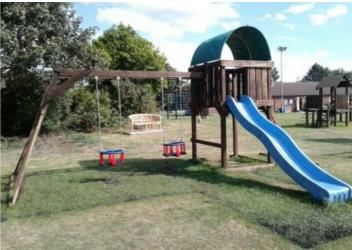
Finding: This equipment has not been designed or installed Action: The equipment should either be removed from use to meet with the requirements of BS EN 1176 for public playground equipment; we have however used our knowledge of these standards to assist in forming the basis of our report.
