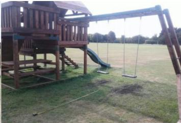
**Finding:** The surfacing dimensions of the monkey bars do not meet with the requirements of the current applicable standard (2.10m required/0.80m provided)
