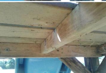
Finding: There are protruding screws beneath the platform Action: Remove the protrusions
