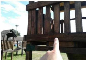
**Finding:** The item fails to meet the requirements of BS EN **Action:** Remove the entrapment 1176 Part 1 4.2.7.2 for head and neck entrapment in the barrier
