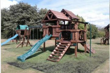
**Finding:** The ramp forms a hard object within the impact area of the slide in contravention of the requirements of BS EN 1176 Part 1
