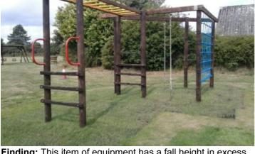
Finding: This item of equipment has a fall height in excess of 2.5m and grass mats have been installed as an impact absorbing surface; these mats rely heavily on the underlying surface to achieve their critical fall height properties.
