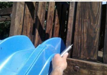
**Finding:** There is/are finger entrapment/s in the barriers and **Action:** Remove the entrapment the item fails to meet the requirements of BS EN 1176 Part 1 4.2.7.6 Entrapment of fingers
