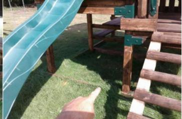
**Finding:** The timber edging forms a hard object within the impact area of the equipment in contravention of the requirements of BS EN 1176 Part 1
