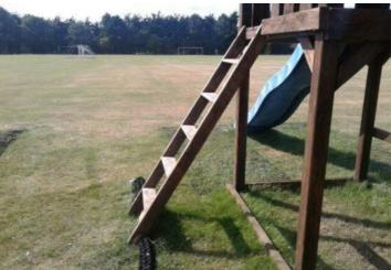
**Finding:** The unit is easily accessible and has an opening in **Action:** Refer to the manufacturer the barrier to steep play elements in excess of 500mm
