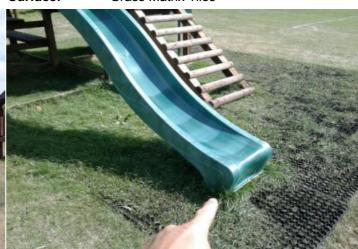
**Finding:** The slide run out is not secured
