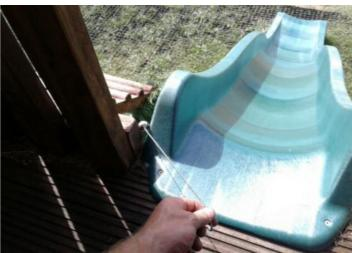
**Finding:** There is a toggle entrapment at the top of the slide, **Action:** Remove the entrapment in contravention of the recommendations set out in BS EN 1176 Part 3
