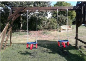
Finding: The lateral stability of the swing seat does not meet with the requirements of BS EN 1176 Part 2; the minimum distance between the suspension members should be the distance between the swing seat connections plus 5% of the suspension length. Distance between crossbeam connections required 44.8cm provided 39cm
