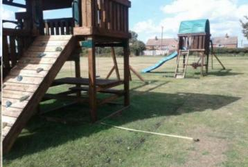
**Finding:** The surfacing dimensions of the platform do not meet with the requirements of the current applicable standard (1.70mm required/1.0m provided)
