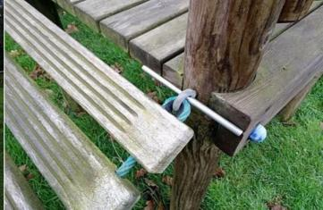
**Finding:** The chain openings are in excess of 8.6mm and do not meet the recommendations of BS EN 1176 Part 1
