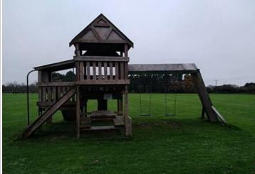
**Finding:** The lower framework forms a hard object within the impact area of the equipment in contravention of the requirements of BS EN 1176 Part 1
