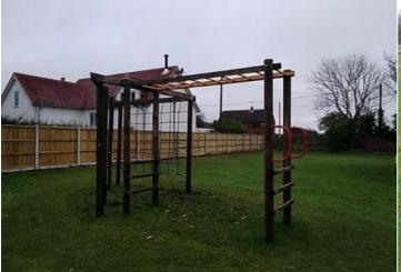
**Finding:** The surfacing dimensions are short and do not meet with the requirements of the current applicable standard
