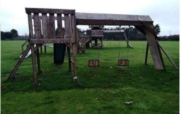
Finding: This equipment has not been designed or installed to meet with the requirements of BS EN 1176 for public playground equipment; we have however used our knowledge of these standards to assist in forming the basis of our risk assessment for the equipment and our report.
