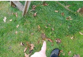
**Action:** Reinstate surrounding surface levels to remove the trip points
