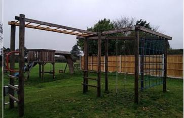
**Finding:** This item of equipment has a fall height in excess of 2.5m and grass mats have been installed as an impact absorbing surface; these mats rely heavily on the underlying surface to achieve their critical fall height properties.
