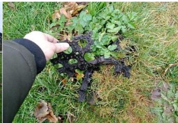
**Finding:** There are damaged sections of grass mass and there are trip hazards present
