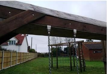
**Action:** We would recommend that the joint be dismantled and checked on a regular basis or a Secondary Safety Device be fitted
