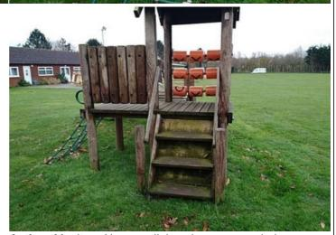
**Finding:** There is an opening in the barriers exceeding the width allowed (500mm) in BS EN 1176, this is a low risk **Action:** Monitor - No remedial work recommended failure and no remedial action is required
