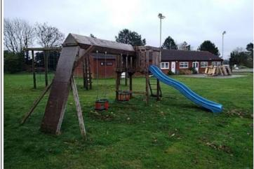
**Finding:** The lower framework forms a hard object within the falling space of the equipment in contravention of the requirements of BS EN 1176 Part 1
